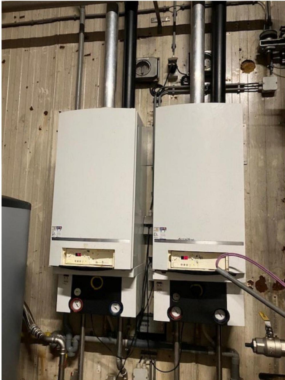
Foto 5: Boilers warmwater
