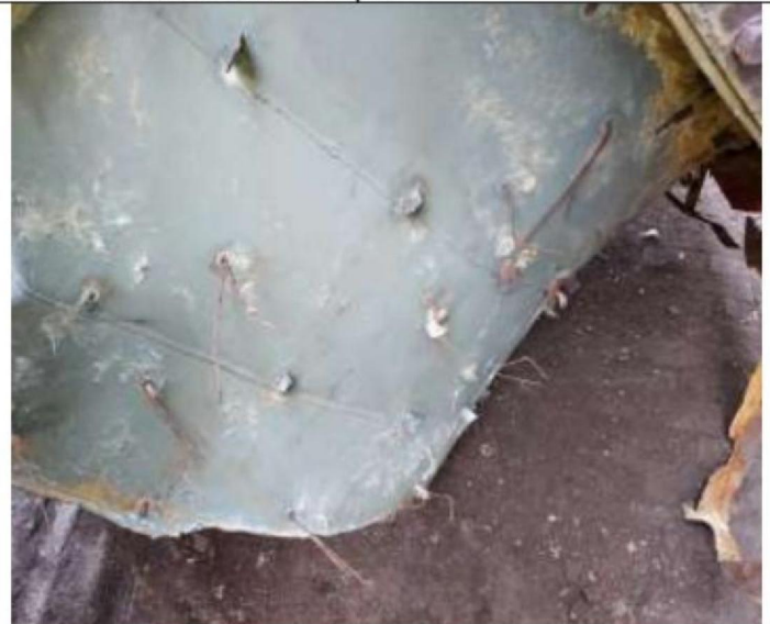
Description photo: 16-3-2021 parts off separation between FGD and Precips
