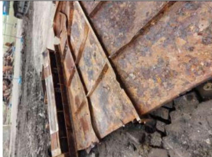
Description photo: 26-3-2021 parts off separation between FGD and Precips
