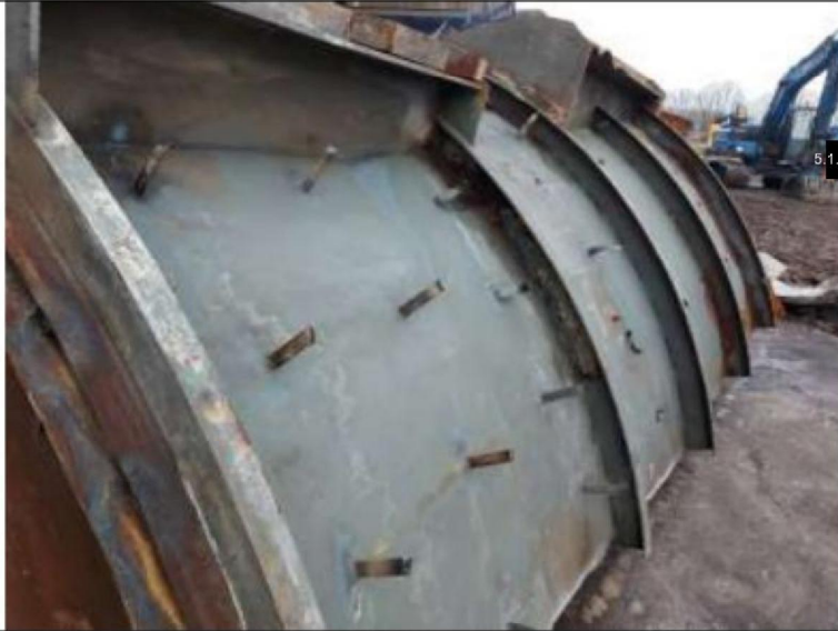
Description photo: 16-3-2021 parts off separation between FGD and Precips
