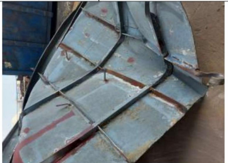
Description photo: 25-3-2021 parts off separation between FGD and Precips
