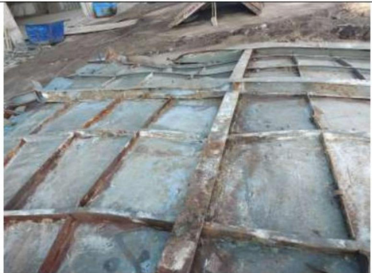
Description photo: 25-3-2021 parts off separation between FGD and Precips
