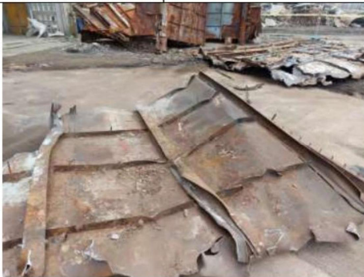
Description photo: 25-3-2021 parts off separation between FGD and Precips
