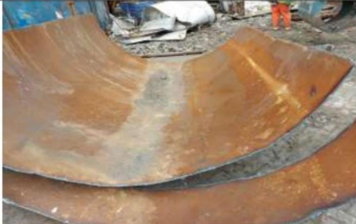
Description photo: 10-3-2021 parts off separation between FGD and Precips
