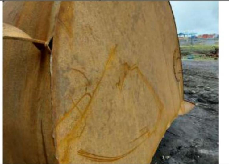
Description photo: 16-3-2021 parts off separation between FGD and Precips
