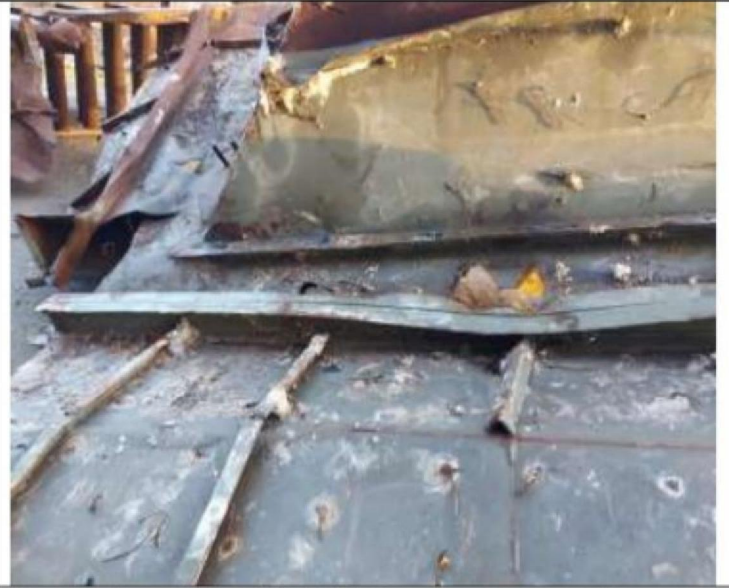
Description photo: 15-3-2021 parts off separation between FGD and Precips
