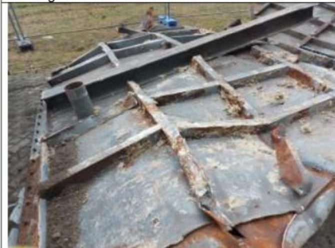
Description photo: 10-3-2021 parts off separation between FGD and Precips
