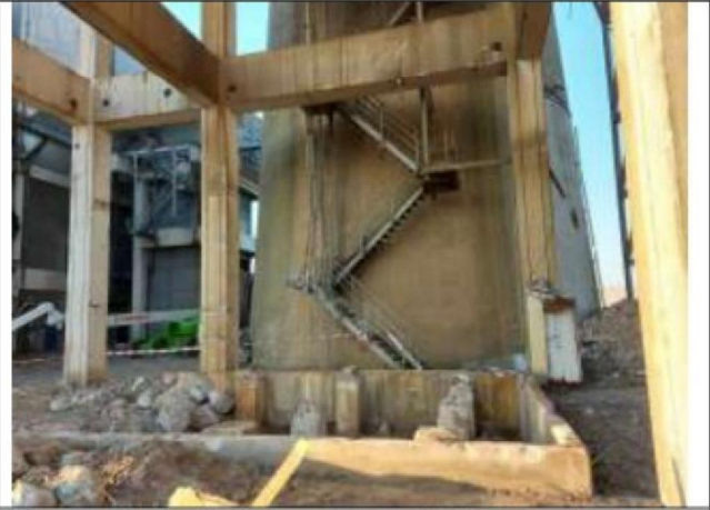
Description photo: position ducts and piping after removal.
