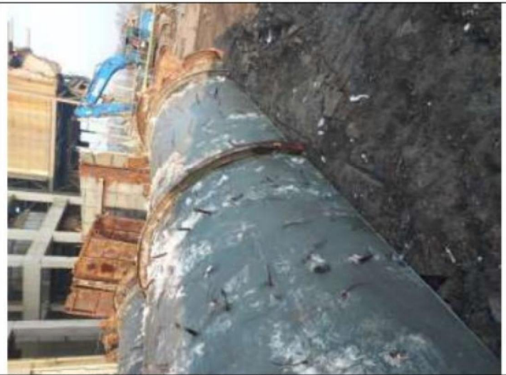
Description photo: 24-3-2021 parts off separation between FGD and Precips
