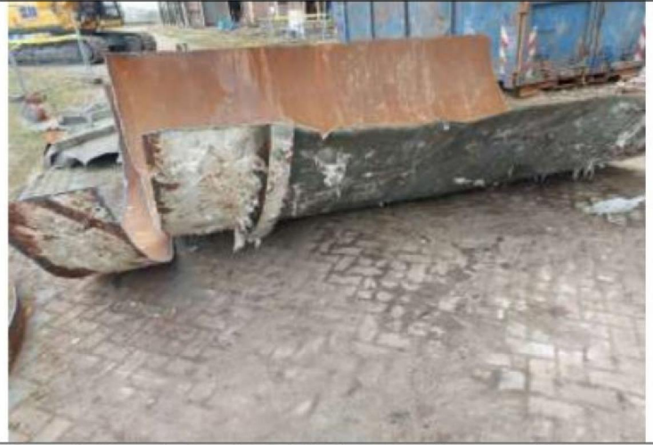
Description photo: 10-3-2021 parts off separation between FGD and Precips
