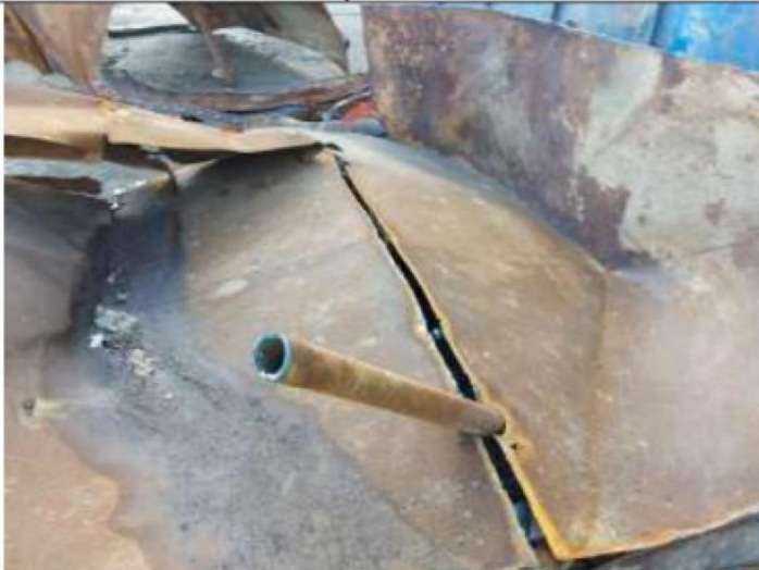
Description photo: 12-3-2021 parts off separation between FGD and Precips
