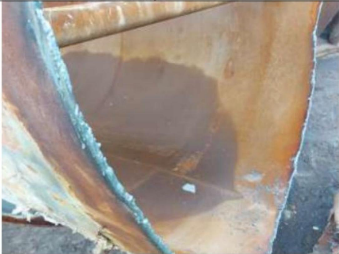
Description photo: 11-3-2021 parts off separation between FGD and Precips
