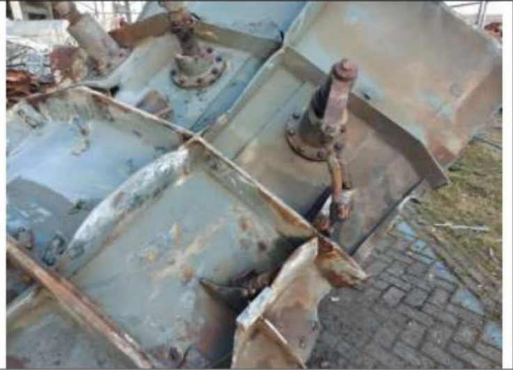
Description photo: 11-3-2021 parts off separation between FGD and Precips
