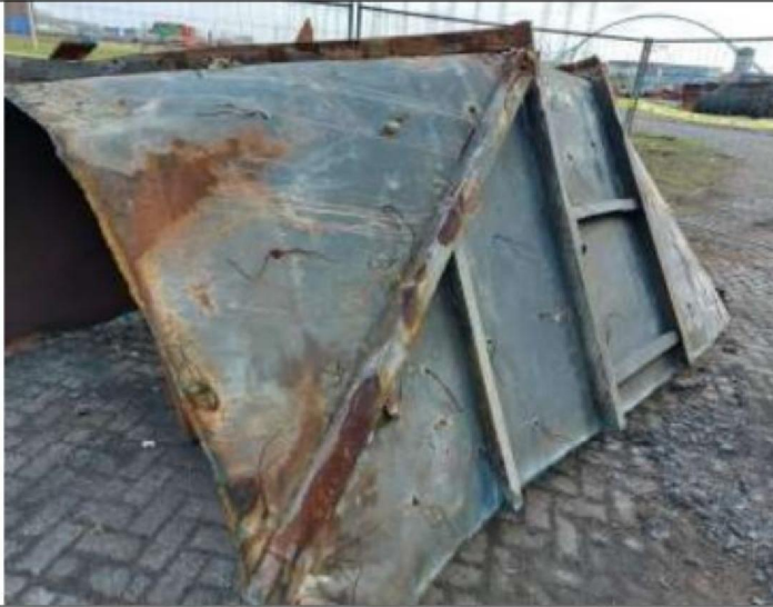
Description photo: 12-3-2021 parts off separation between FGD and Precips
