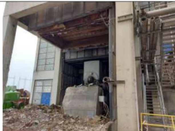
Description photo: position ducts and piping after removal.
