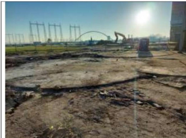
Description photo: clean concrete floor after removed the asbestos stamps and textile bandage
