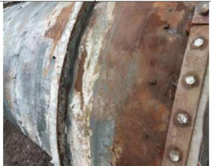
Description photo: 17-3-2021 parts off separation between FGD and Precips
