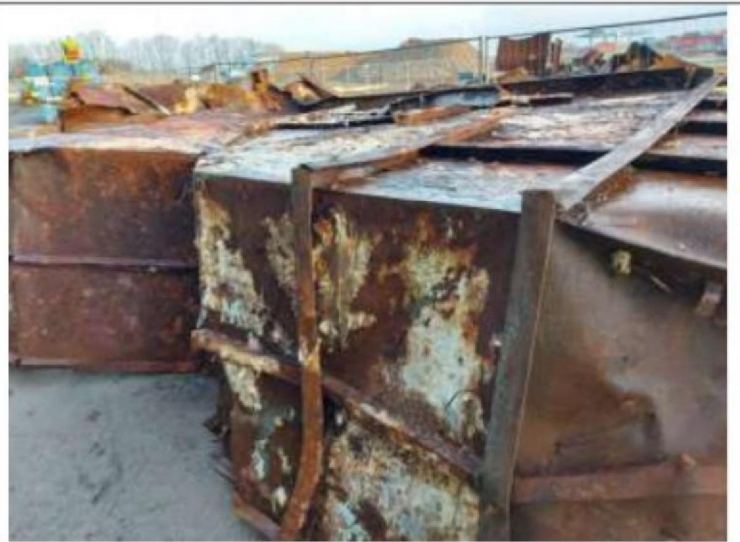
Description photo: 15-3-2021 parts off separation between FGD and Precips
